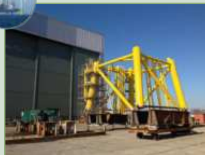
SUPPORT PRE-ASSEMBLY SURVEY
